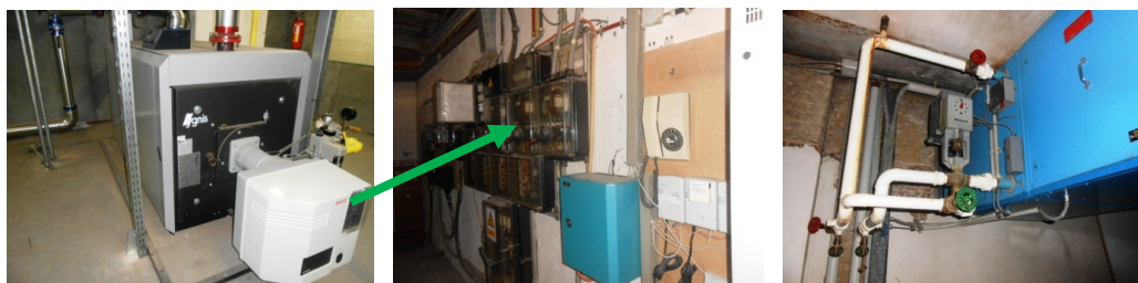
photo: 4, installation technique
