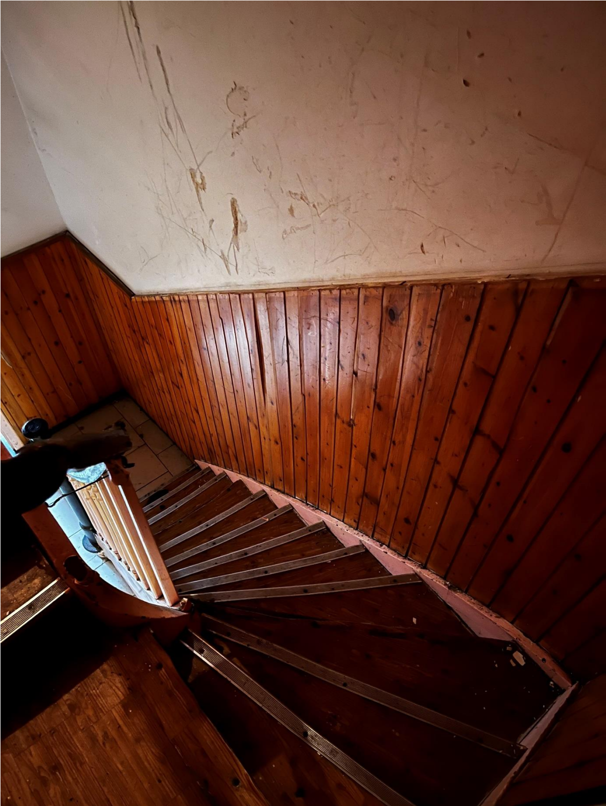
Escaliers menant aux diverses parties privatives
