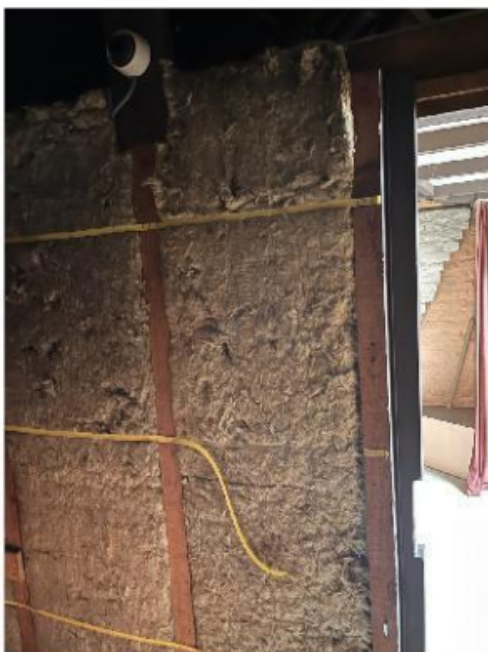
isolation cloison grenier
