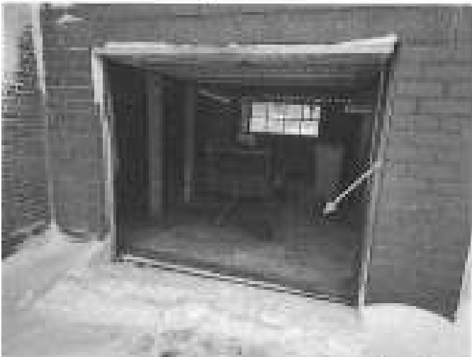
ruwe beton / chape
