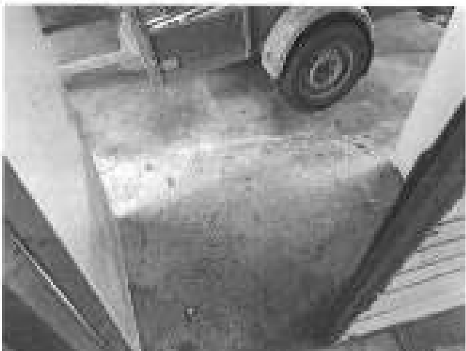
ruwe beton / chape
